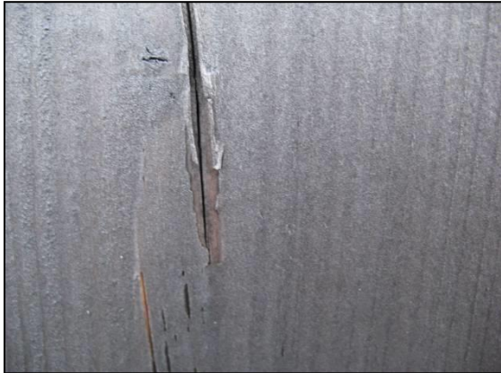
Fig. 2.2: Crack formation and flaking
