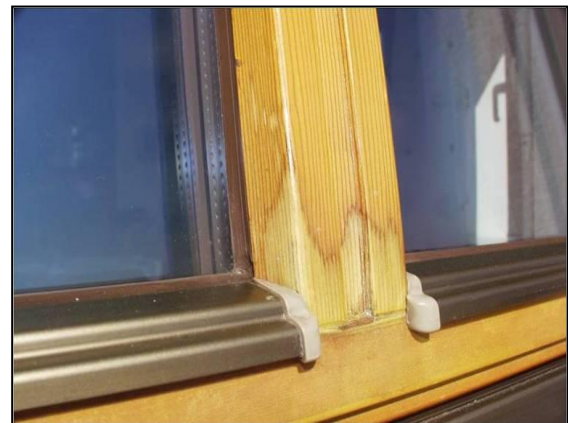
Fig. 4.6: damage in the joint area
