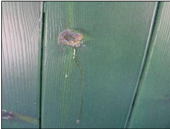
Fig. 2.4: Bleeding of resin in the knot area
